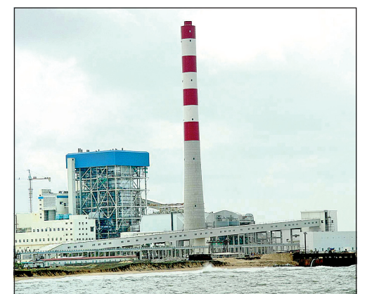
The Norochcholai Thermal Power Plant to meet the soaring power requirement of the country
