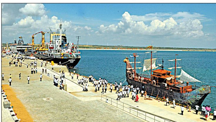
The Magampura Mahinda Rajapaksa Port which was constructed inland, the first of its kind in the world
