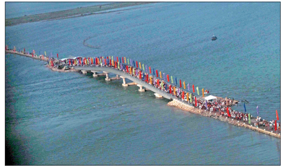
The Sangupiddy bridge shortening the distance between the South and North
