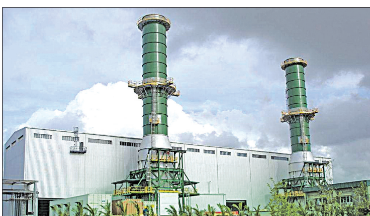
The Kerawalapitiya thermal power plant to energize the government's aim of electricity for all
