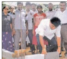
The Panadura Public Housing Development Fund with public donations is constructing a house for war hero, Lance Corporal B Ashan Aravinda Mendis. Here Public Housing Development Fund convener Sandipa Radella laying the foundation for the house. Picture by Geetha de Mel
