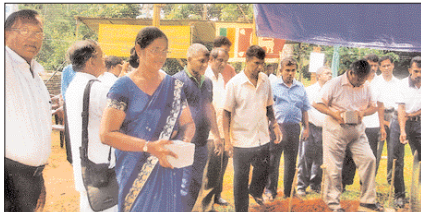
Peoples Bank Manager Baddegama Asoka Mawellage and the Opposition Leader Baddegama Pradeshya Sabha Ananda Lanerolle laid the foundation stones for the construction of a memorial for war heroes at Baddegama recently. Former Southern Provincial Council member Ananda Abeywickrema was also present. Picture by Somadasa Abeywickrema, Baddegama Group Correspondent
