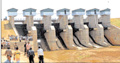
The President inspecting the shutters of the dam
