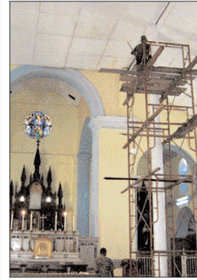
Repairs inside church
