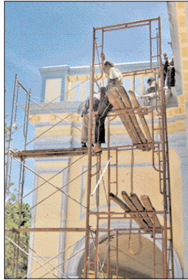
Work in progress outside
